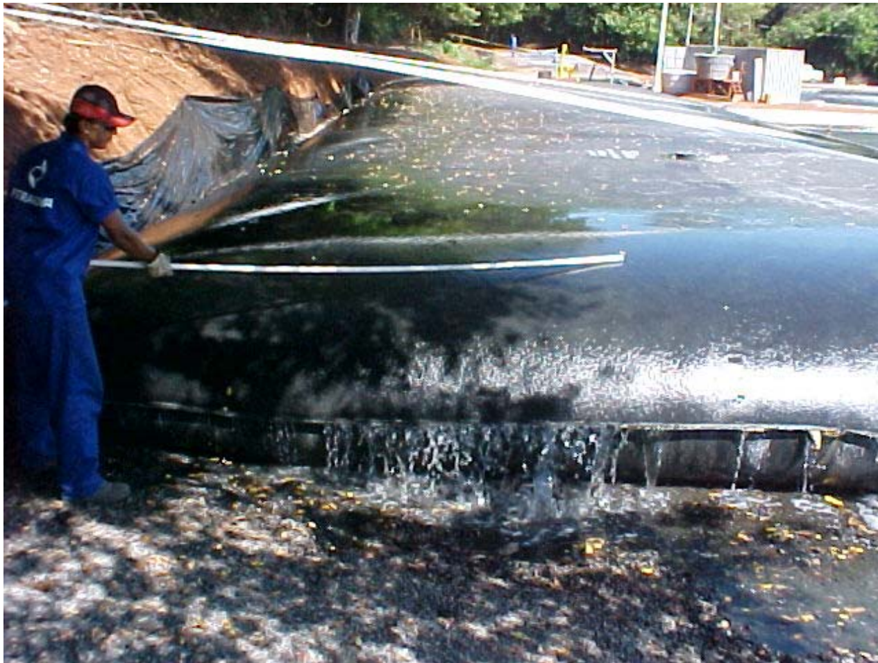
Photo 3: BAG full of mud in the process of dehydration
